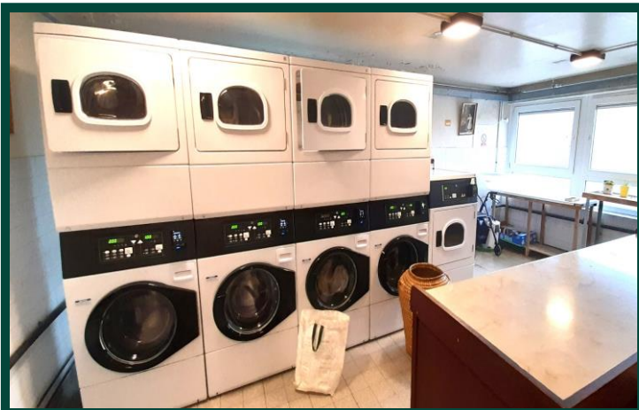
Communal Laundry Room
